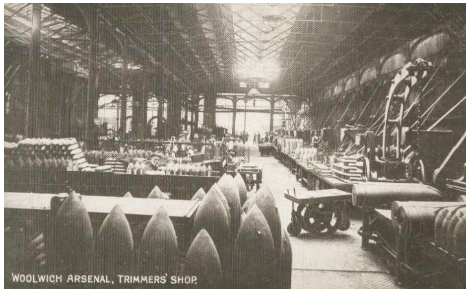
Trimmers' Shop Woolwich Arsenal. (All photos were added to original story)
