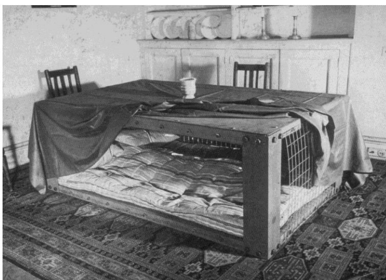
Indoor Morrison Air Raid Shelter doubles as a table.
