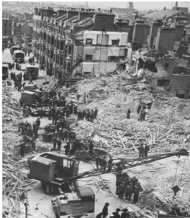
WWII bomb damage.
