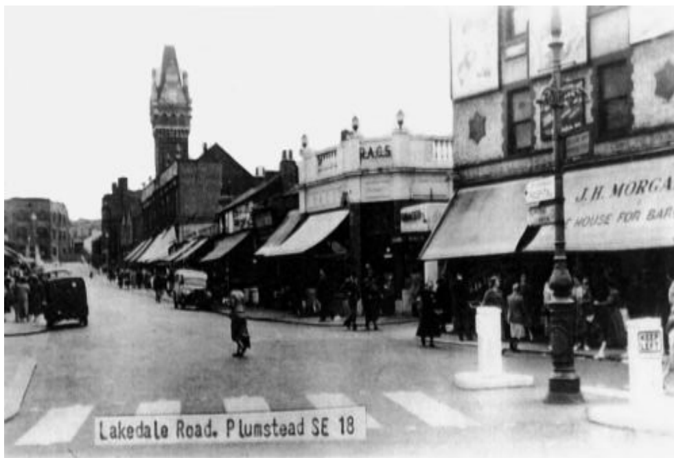
Lakedale Road, Morgan's' shop is on the right. Photo: Alan Gibbs.
