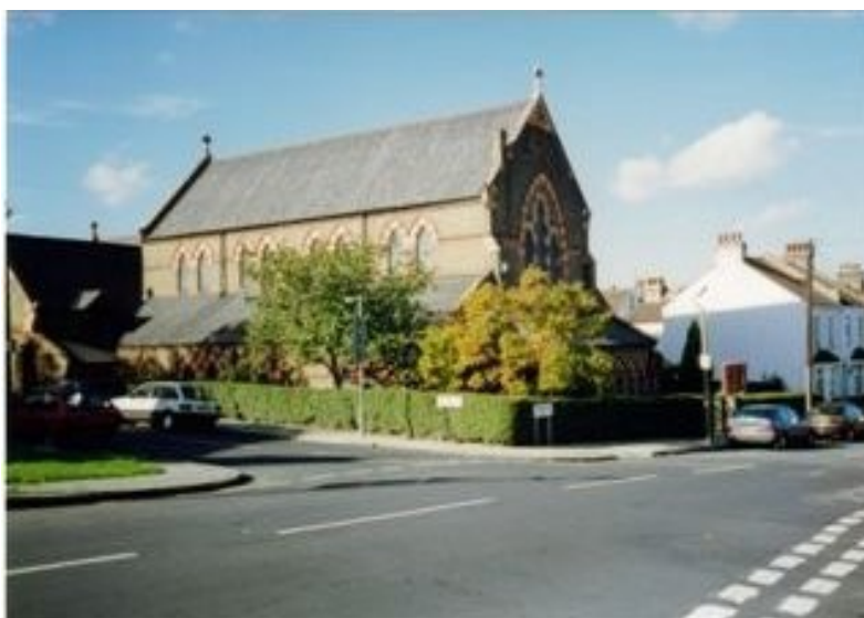
Ascension Church, Timbercroft Lane, adjacent to the school.
