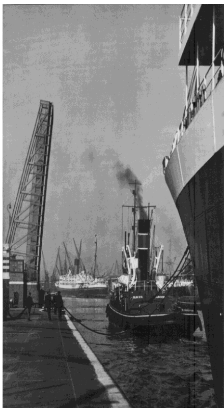
Road drawbridge is up as a ship enters the KGV Docks. Photo: RS Rawlings 1950.
