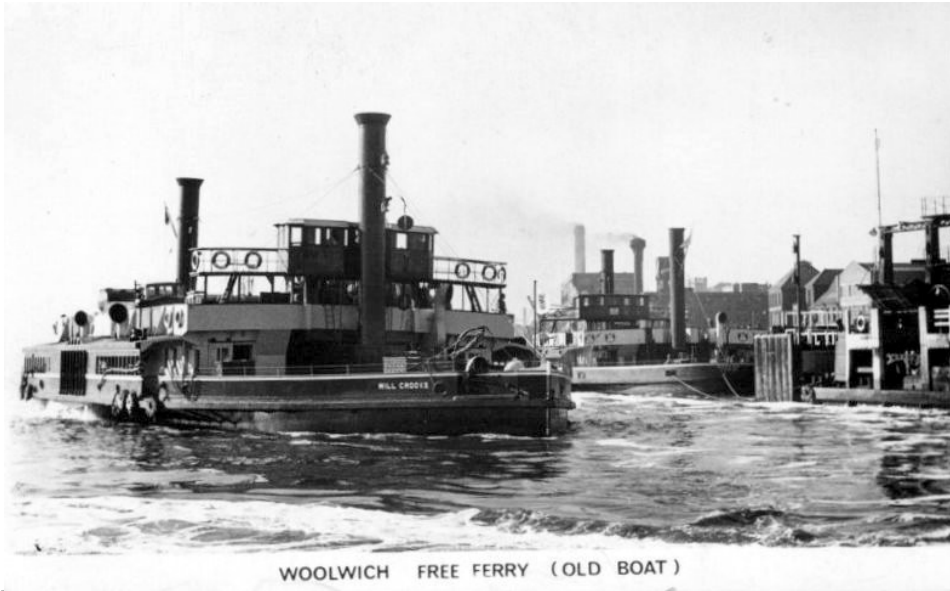
The old Woolwich Free Ferry. (Southern Approach)
