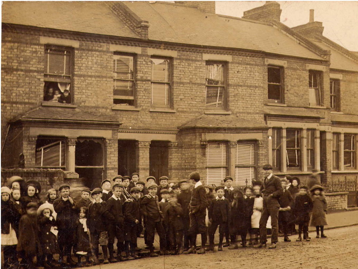
Gas Explosion Damage, Reidhaven Road, Plumstead, 11-2-1907, in the early Edwardian era. Photo: Beverly Bryant, taken she thinks by her grandfather William Driver.
