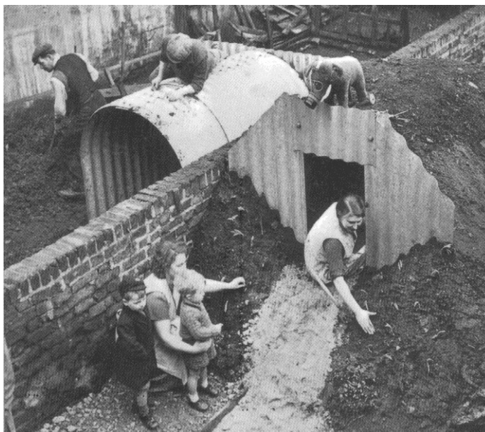
Families installing their Anderson air raid shelters in their back gardens.
