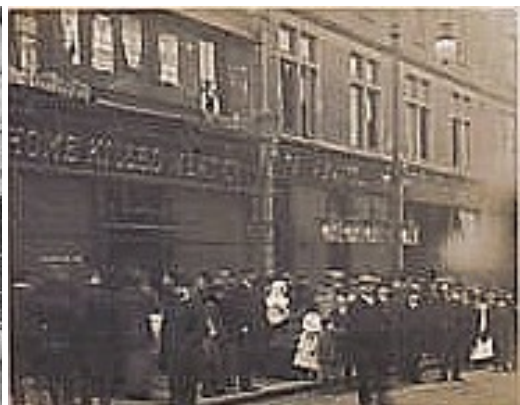
High Street shop damage from gas explosion.
