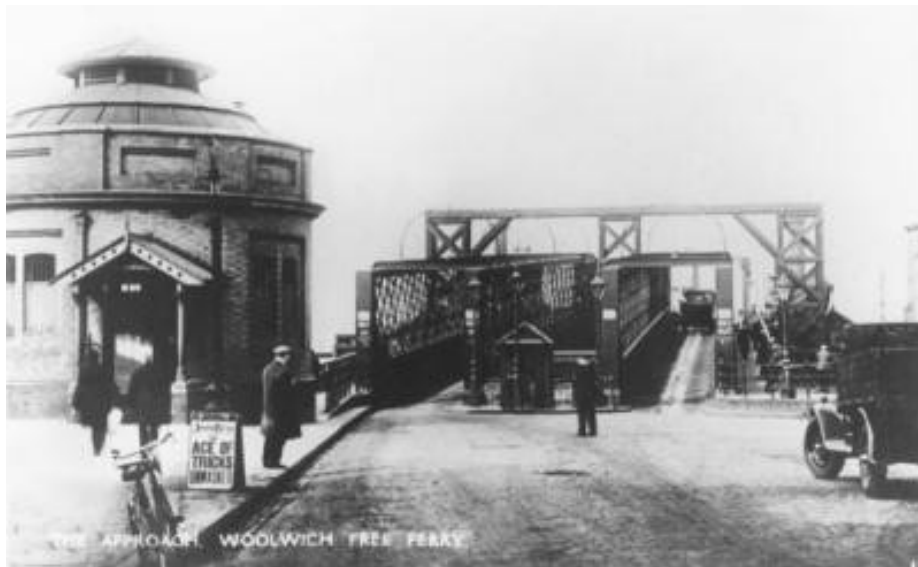
The old Woolwich Free Ferry approach road ramps, south side.
